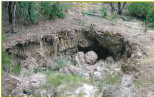
Figure 5. Piping failure or tunnel erosion in a dam constructed from soils derived from Permian mudstone. This dam is known to have failed on first filling. The image was taken from the dam floor.
