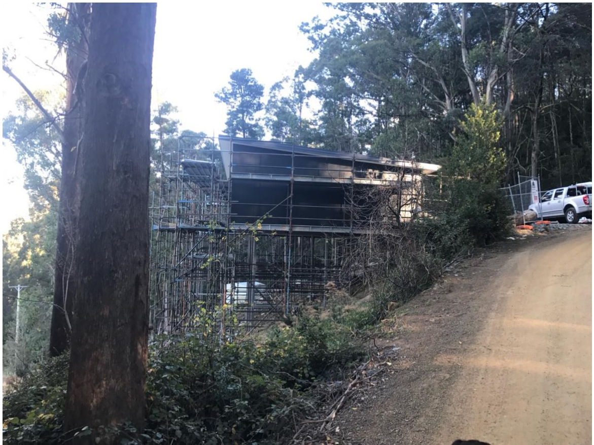
East of property during construction 2019 with bank entirely overgrown with Ilex Aquifolium and Rubis Fruticosus
