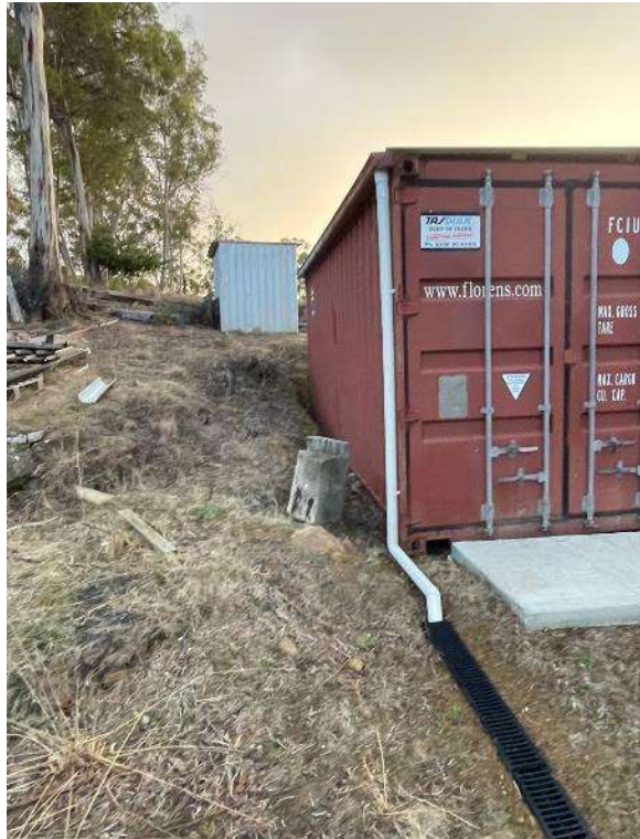
Photo 5: Looking north along western elevation of subject structure. Note excavation, roof drainage, and grated surface drain.
