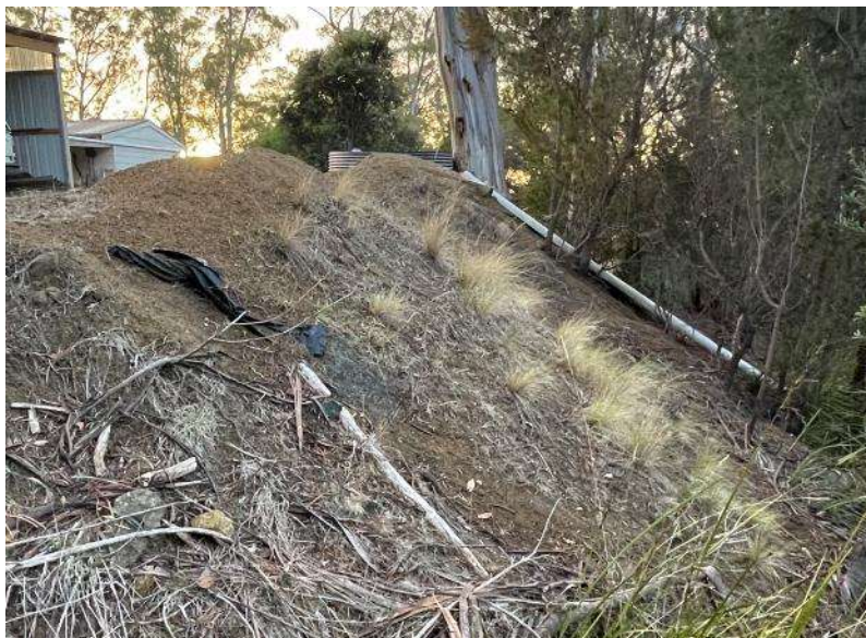
Photo 4: Western end of fill looking east.
