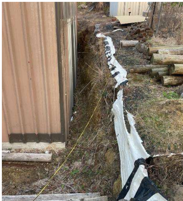
Photo 6: Looking west along northern elevation of shipping container/lean-to. Note excavation.
