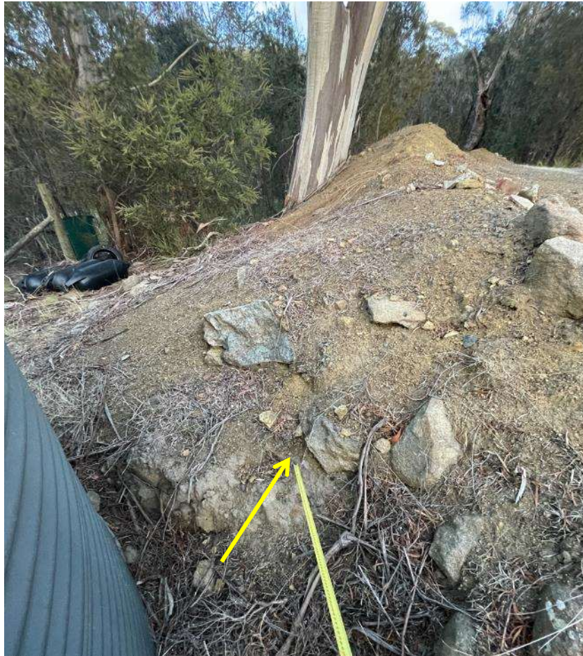
Photo 3: Eastern end of fill looking west. Previously existing/natural ground can be observed.
