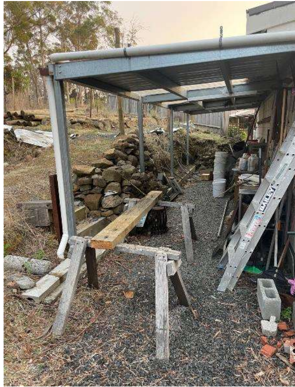
Photo 7: Nearby excavation along western elevation of adjacent shed/garage.
