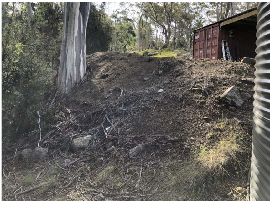
Photo 2: Eastern end of subject fill viewed from downslope.
