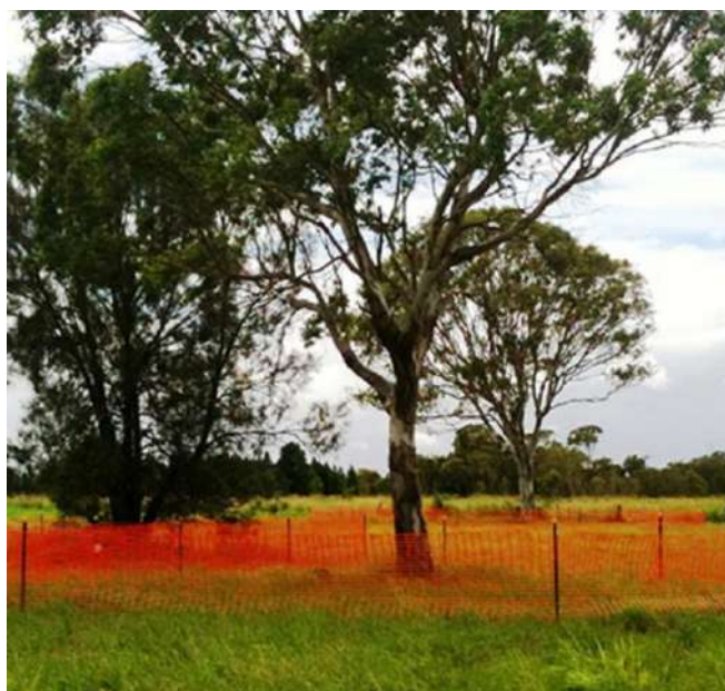
Figure 8- Tree Protection Fencing constructed with barrier mesh.
