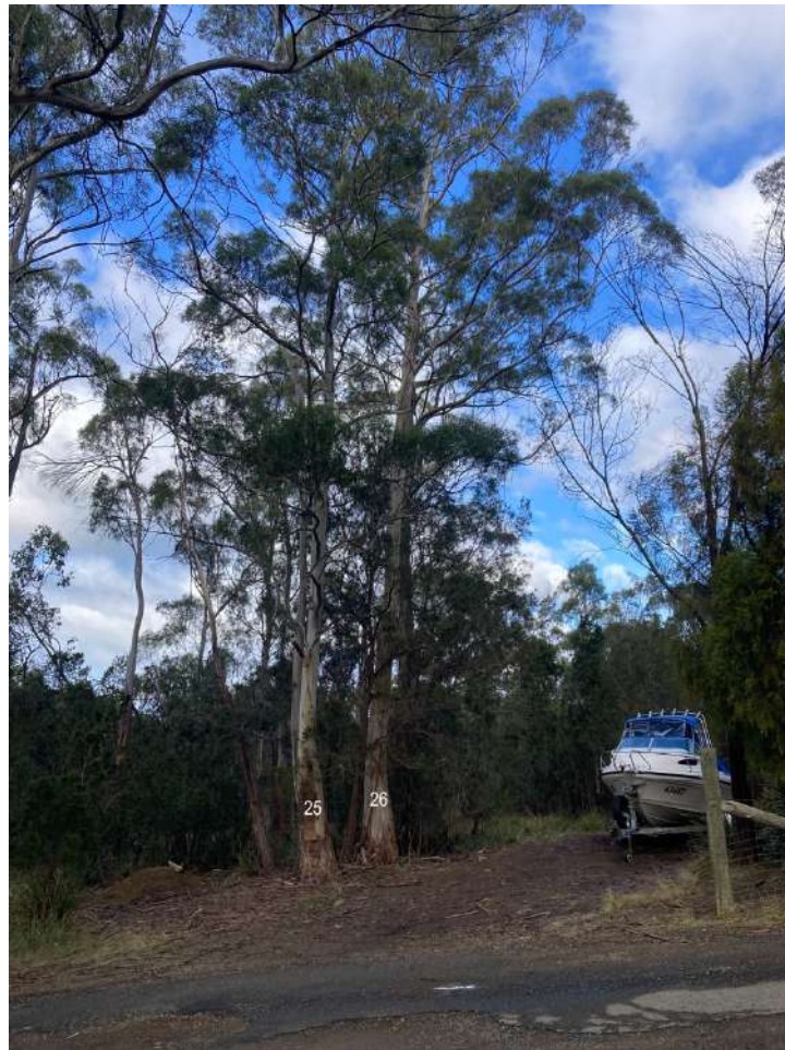
Figure 5: The fill deposit & compaction for construction of the boat parking/storage area in the root zones Of trees 25 & 26
