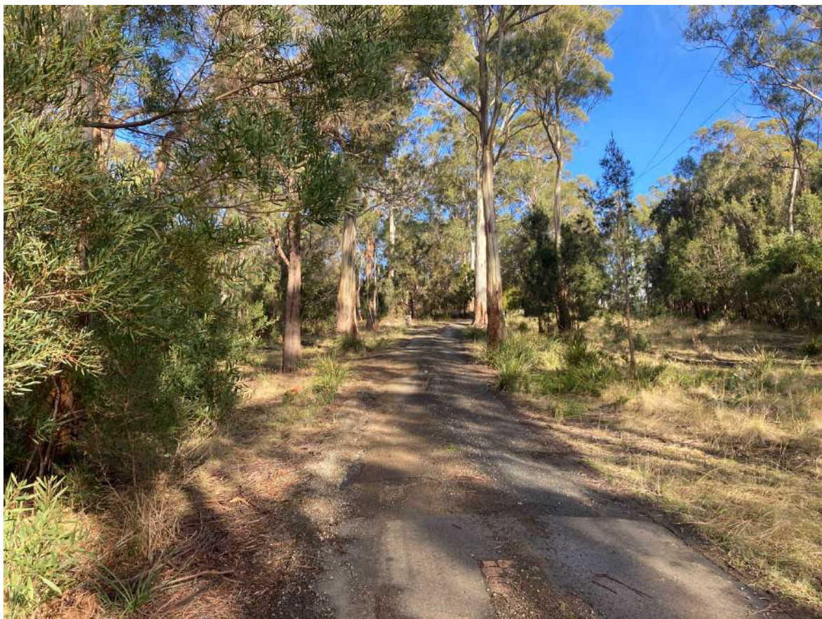
Figure 2: The existing access lower section looking southwest from the start of the survey area at chainage ~65m to chainage 120m (approx.)
