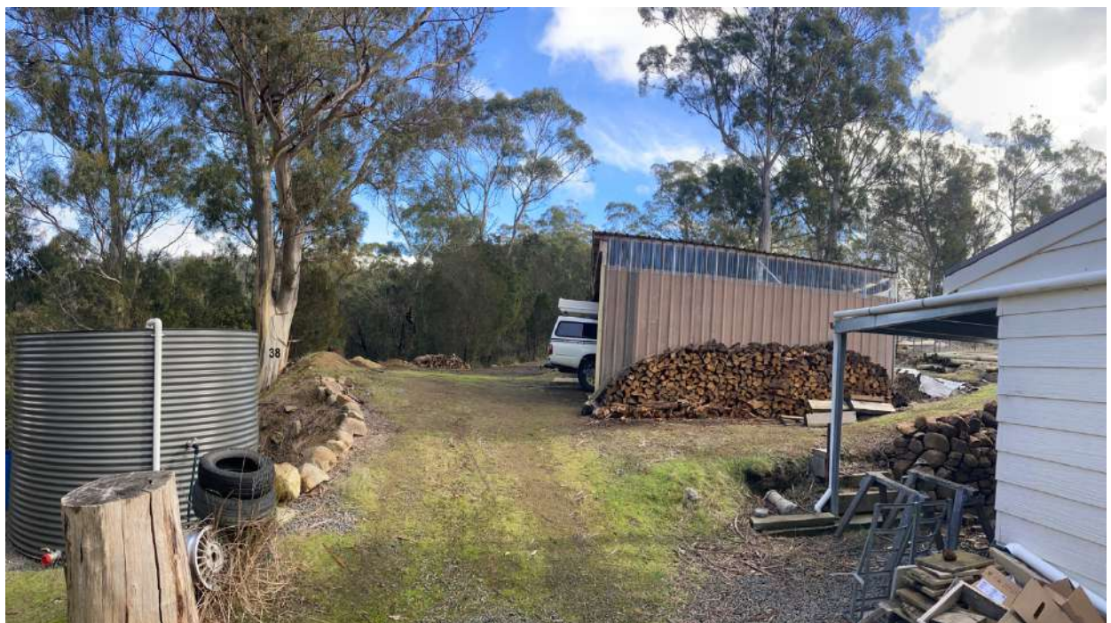
Figure 4: The area of bulk earthworks associated with the subject outbuilding/lean-to in the root zone of tree 38
