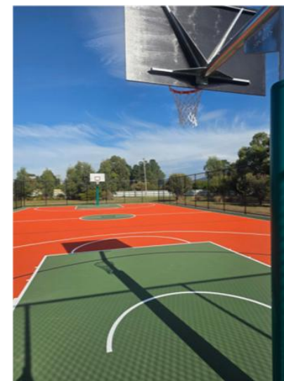
Basketball Courts at Dru Point, Margate
