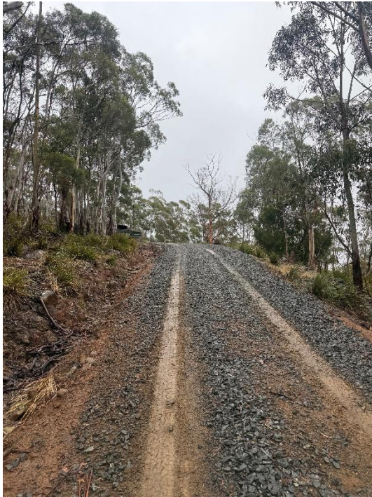
Figure 7. Image of above grade access road.
