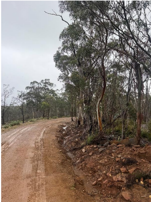
Figure 3. Image of above grade access road.
