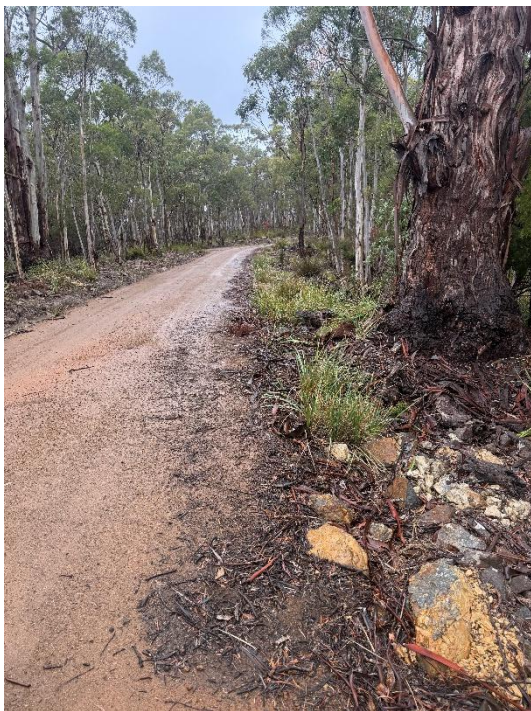
Figure 5. Image of above grade access road.
