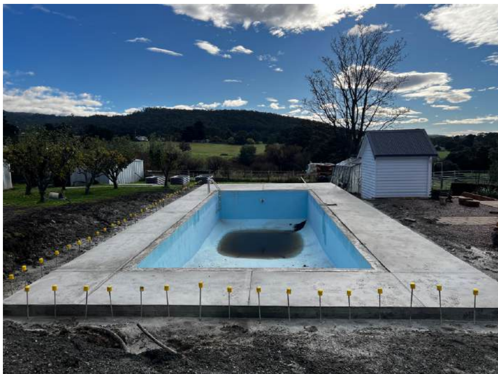
Image 12: Existing pool (Photo taken on site 30/5/2026)
