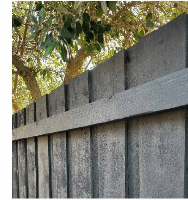
FEXG01 - EXISTING TIMBER PILING FENCE 1800 HIGH
