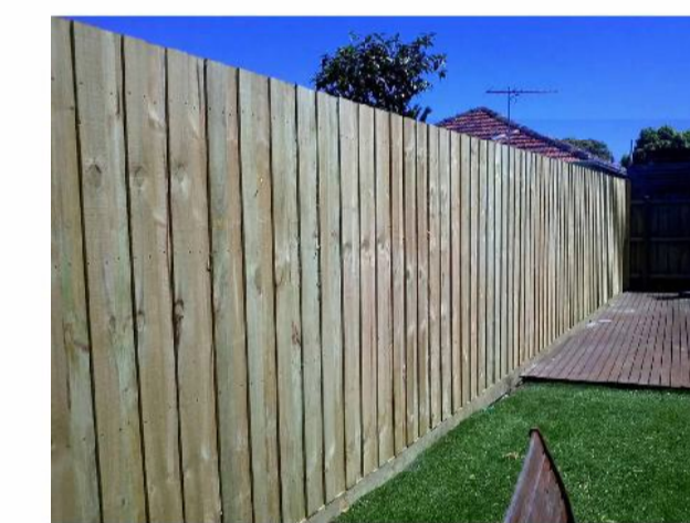
F02 - TIMBER PILING FENCE 1800 HIGH
