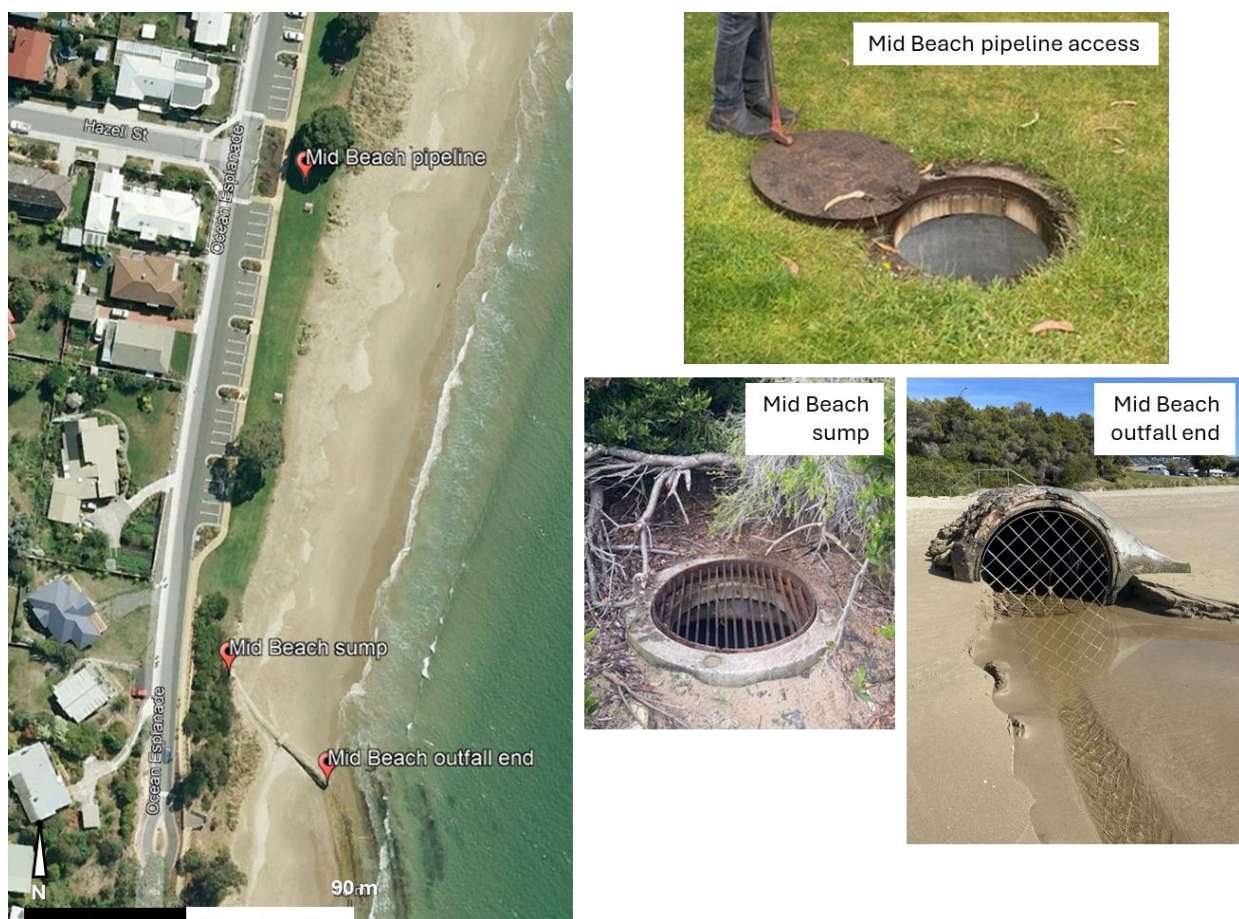
Figure 20. The Mid Beach outfall, showing location of the access point on Ocean Esplanade opposite Hazell Street (Kingborough Council Mid Beach stormwater sampling point), location of sump and the outfall end on the beach.
