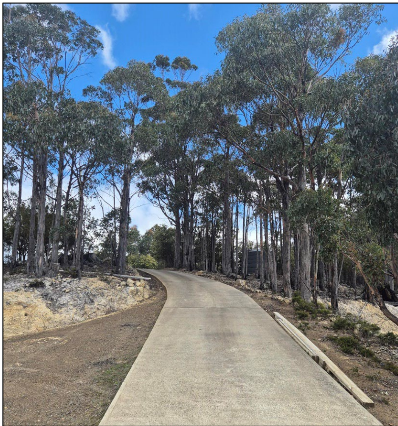
Plate 5: Existing concrete driveway to existing residence
