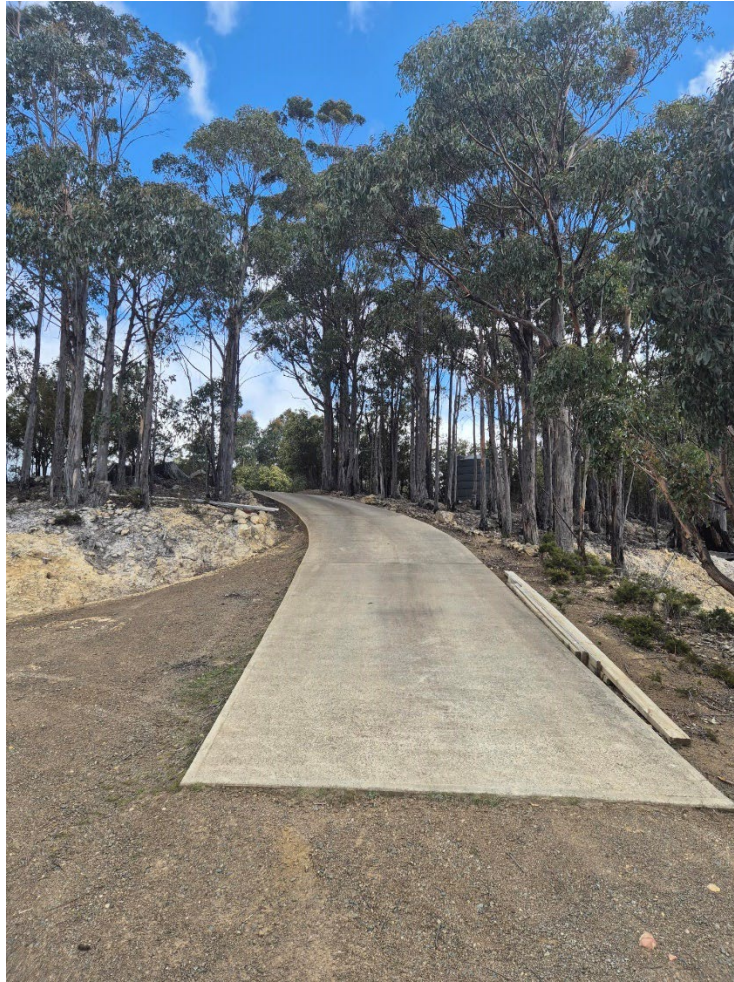
Photo 5 – Existing concrete driveway on slope >10^\circ (<30m to Van Morey Road).
