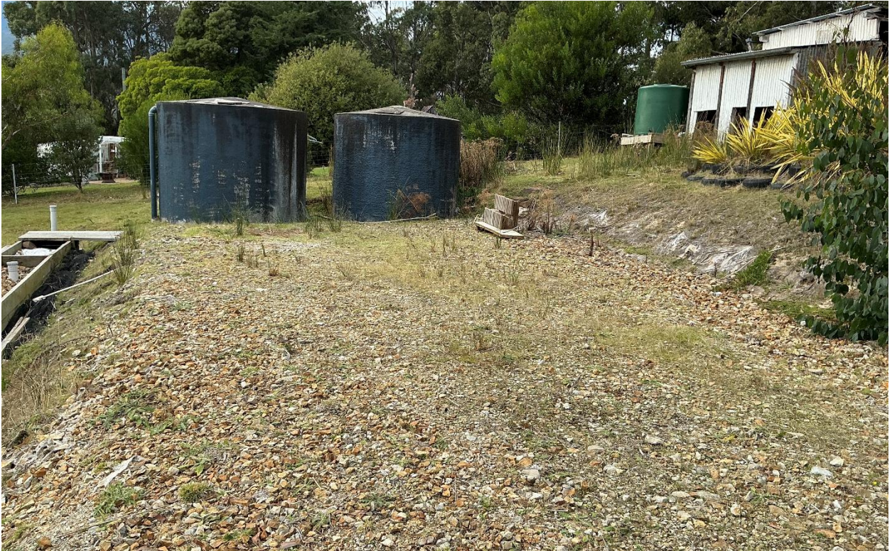
Photo 1 Gravelled lower/middle bench area with water tanks visible downslope. The photograph shows the relatively level pad area and provides context for the cut/fill transition located upslope toward BH01.
