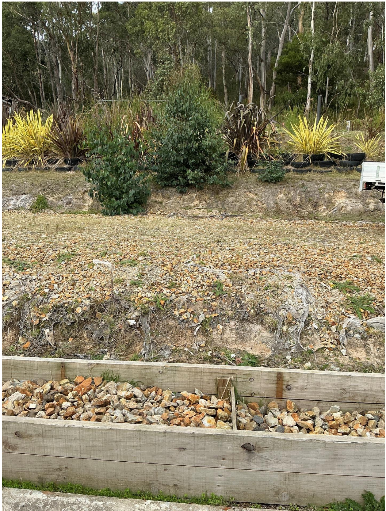
Photo 4 View of the cut/fill face between the upper and lower bench areas, with the lower retained gravel area in the foreground. The photograph shows the earthworks and batter geometry upslope of the lower bench.
