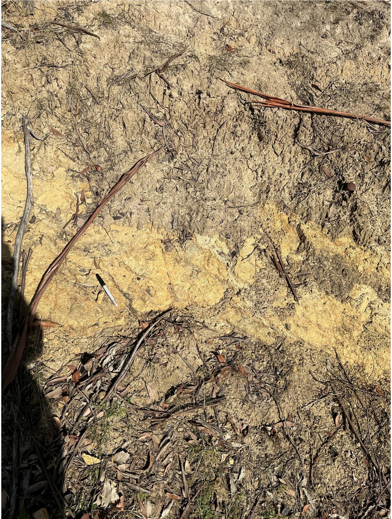
Photo 5 Close-up of exposed soil/weathered material within the cut batter of the upper bench, showing the nature of the near-surface materials encountered in the historical earthworks area.
