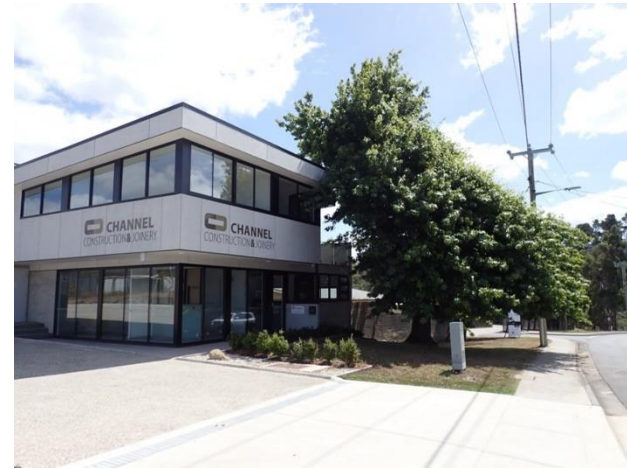
Figure 3. The oak's root zone and crown have been impacted by historic construction and pruning for clearance from electrical conductors.
