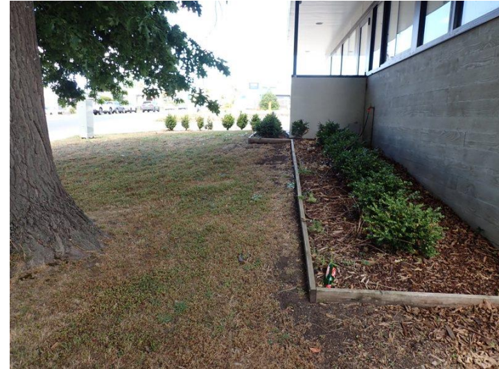
Figure 5. The path extension (footprint approximates the extent of the edged garden bed) has potential to impact on structurally significant roots extending toward the building.
