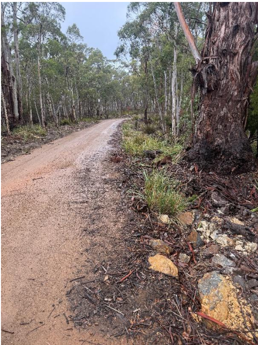
Figure 5. Image of above grade access road.
