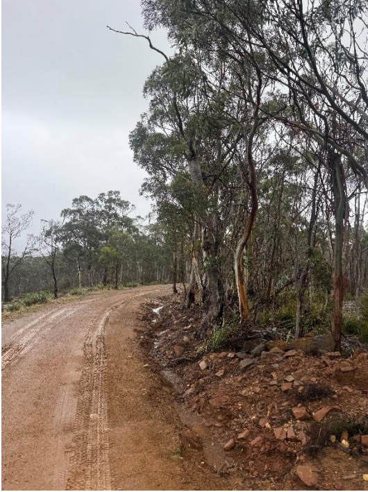
Figure 3. Image of above grade access road.
