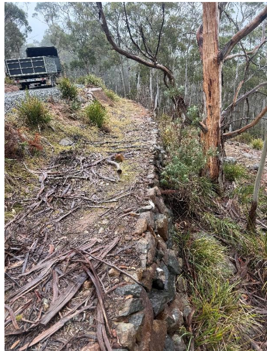
Figure 6. Image of old stone wall separating trees and access road.
