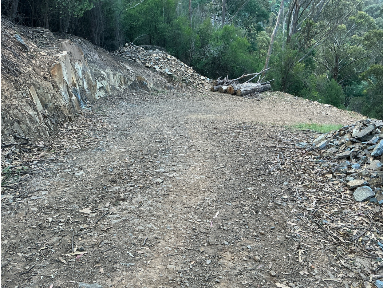
Photo 5 Evidence of exposed slightly weathered dolerite bedrock on the northern section of the driveway
