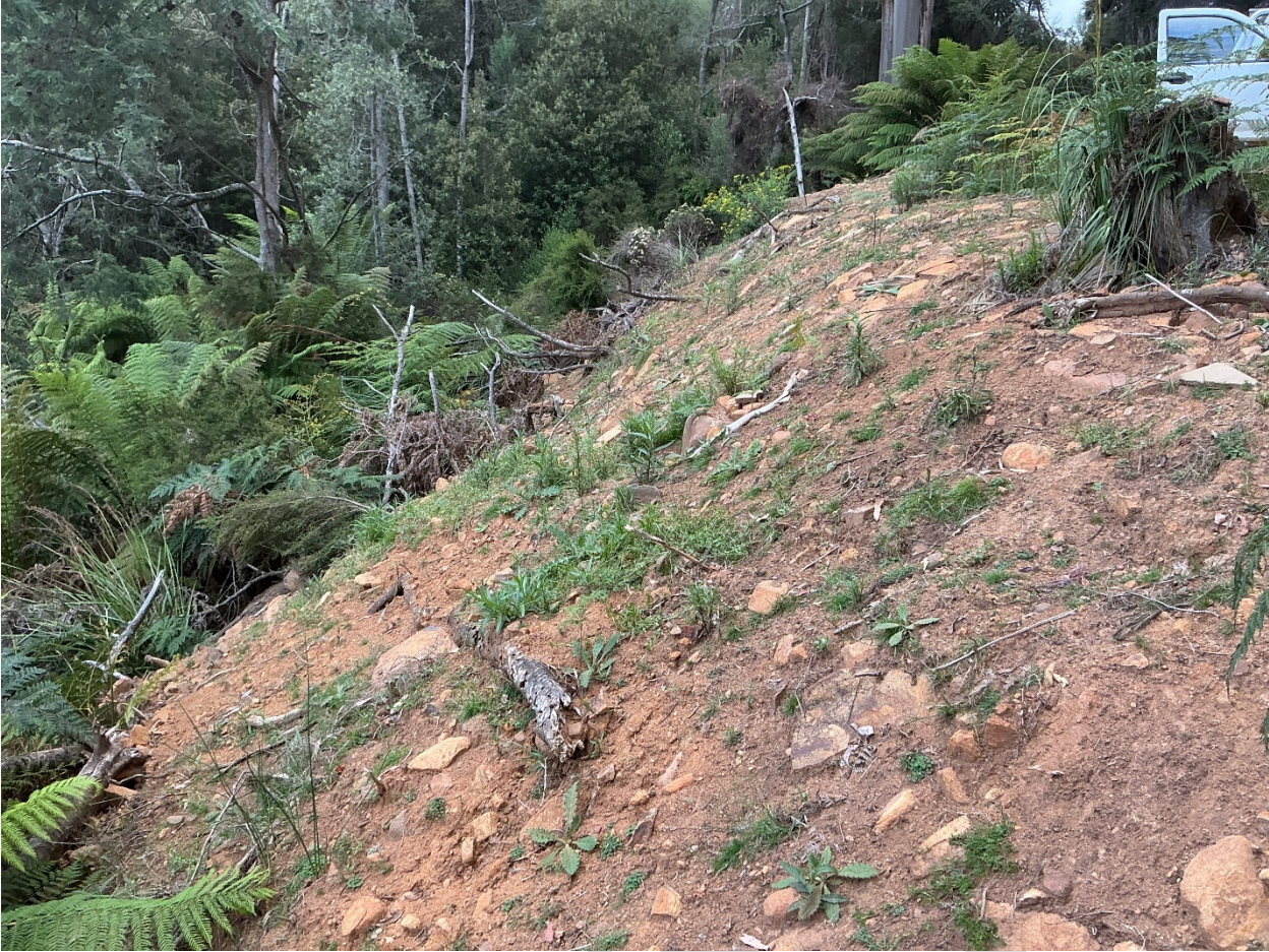
Photo 7 Overview of road fill area
