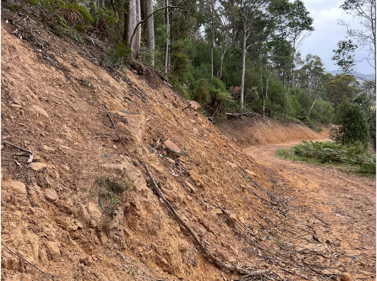
Photo 3 Colluvium deposits in the existing road cut.
