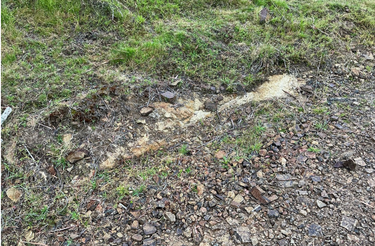
Photo 1 Evidence of exposed dolerite bedrock on the lower section of the driveway
