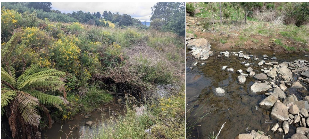
Figure A4.6-2 Cooke's Rivulet in the vicinity of the current bridge, has very little native aquatic or riparian vegetation
