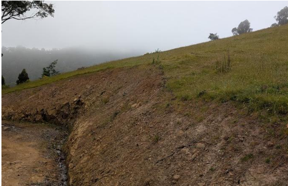
Figure 5.2-4 The fourth corner of the access track will require widening to meet BAL requirements, no vegetation clearance is required.
