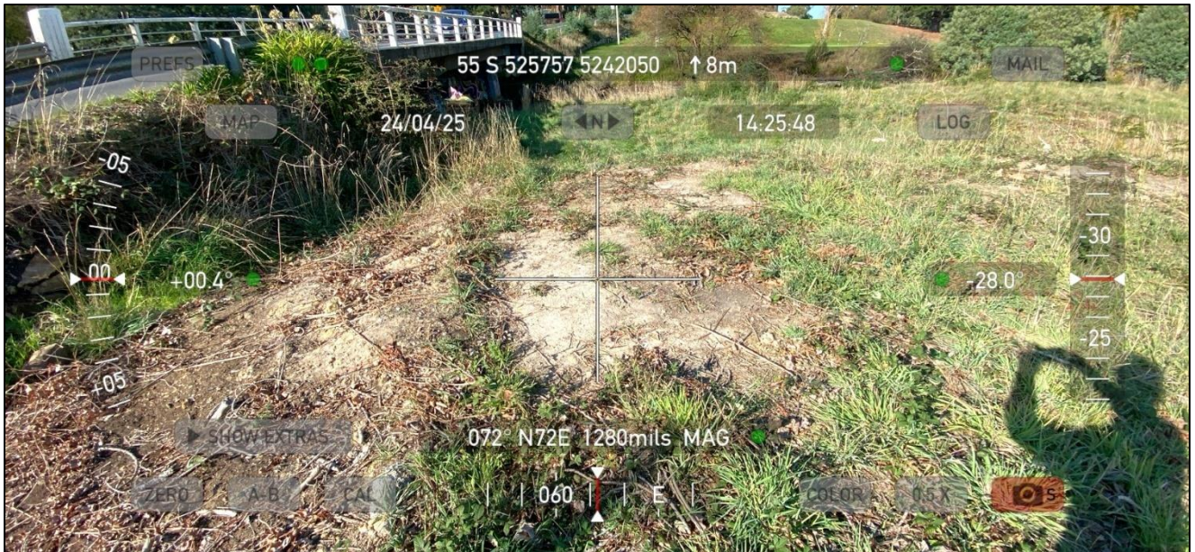
Figure 28 - Location where drilled line under Browns River started (approximately 20 m from rivers edge)
