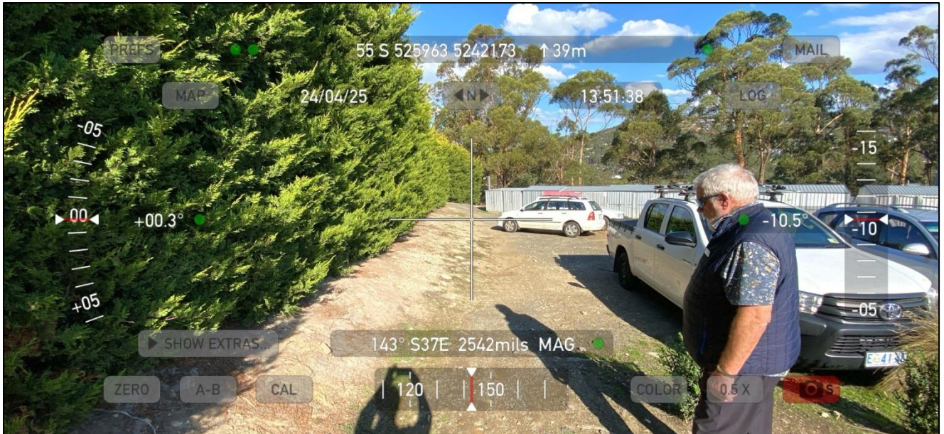
Figure 14 - Alignment of new sewer line beside the carpark of the Golf Club
