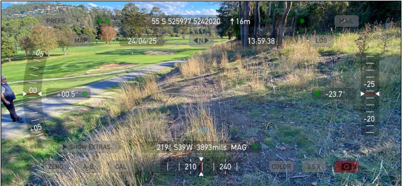
Figure 19 - Alignment of new sewer line where it passes close to remnant DGL forest at left
