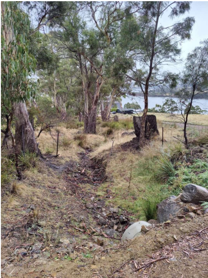
Figure 21 Existing culvert and natural creek
