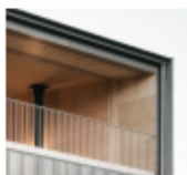
Balustrade + timber walls
