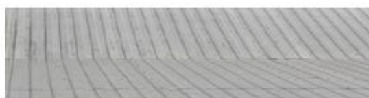
Weathered Zinalume — matte, uniform grey
