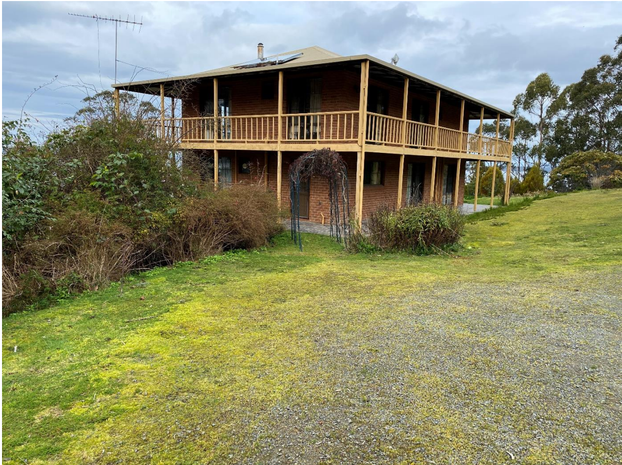
Figure 5 Looking SE at The existing dwelling.
