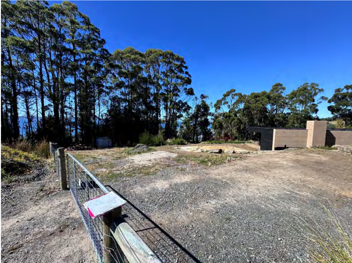
Side & rear of existing structure to right, site of extension ahead
