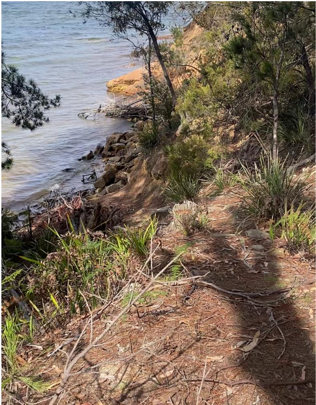
Figure 14 – View from the existing pathway showing the location of the landward end of the proposed jetty and the section of the existing pathway to be upgraded (Kingborough Council).
