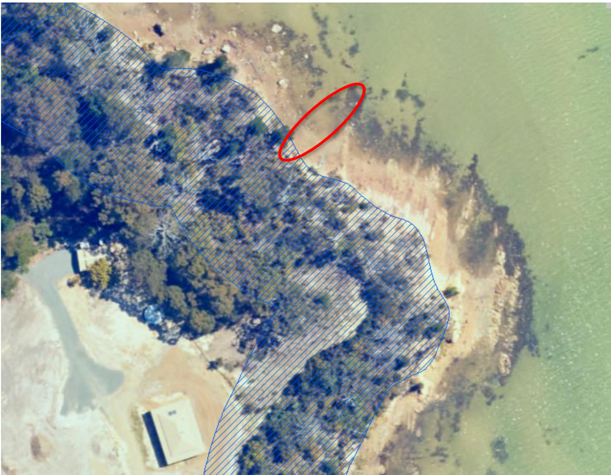
Figure 5-1 – Kingborough Interim Planning Scheme - Waterway & Coastal Protection Area (Source: Listmap)
