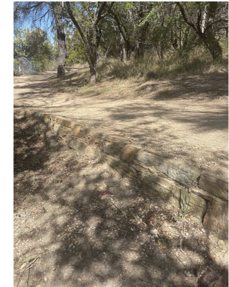
Mudstone rock to be placed at edges to retain gravel where needed and to help reduce erosion. Shallow, rock paved gutters to be provided across the path where the natural runoff indicates.
