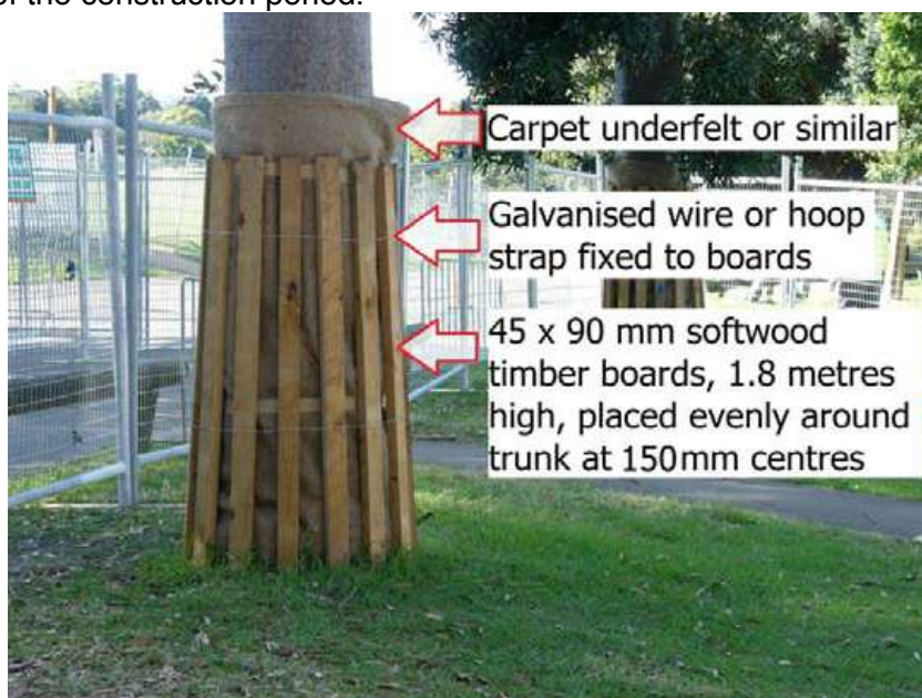
Figure 12- Example of tree trunk protection
