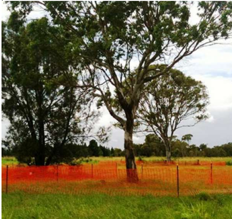
Figure 10- Tree Protection Fencing constructed with barrier mesh.
