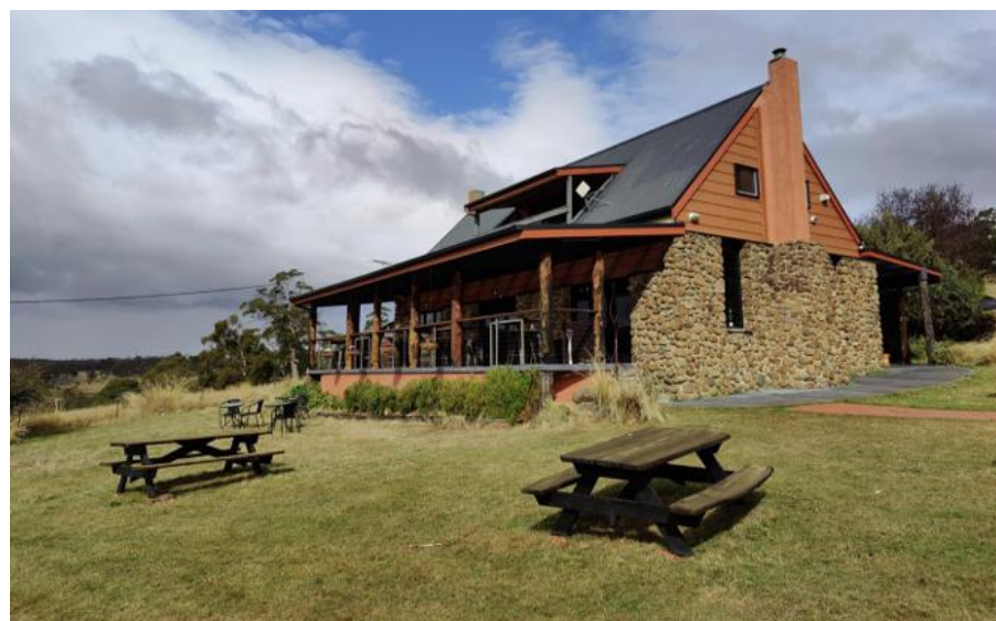
Figure 7: View of Bruny Island House of Whisky from the outside (source: TIA prepared by GHD)
